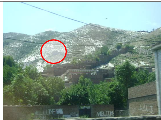
Gravity fed water scheme: water tanks (circled red) are often in open though fairly difficult to reach areas. The pipes run down the hill above ground and thus are prone to damage/theft.
