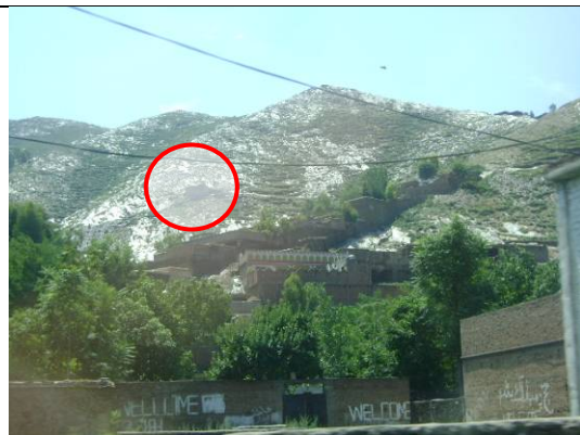
Gravity fed water scheme: water tanks (circled red) are often in open though fairly difficult to reach areas. The pipes run down the hill above ground and thus are prone to damage/theft.
