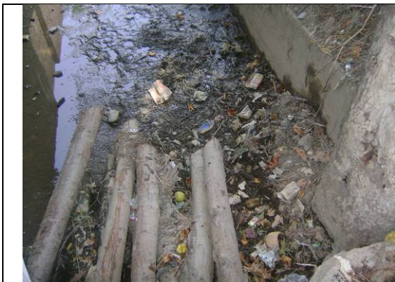
Clogged drainage as a result of waste being improperly disposed of.
